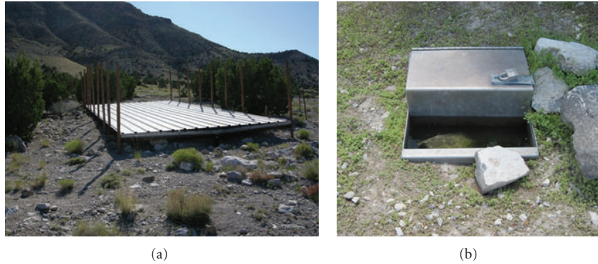
FIGURE 1: Typical wildlife water development on the Thomas-Dugway Mountains in western Utah, USA, including catchment apron (a) and drinker (b) where we photographed mule deer using water sources, 2007–2011.
